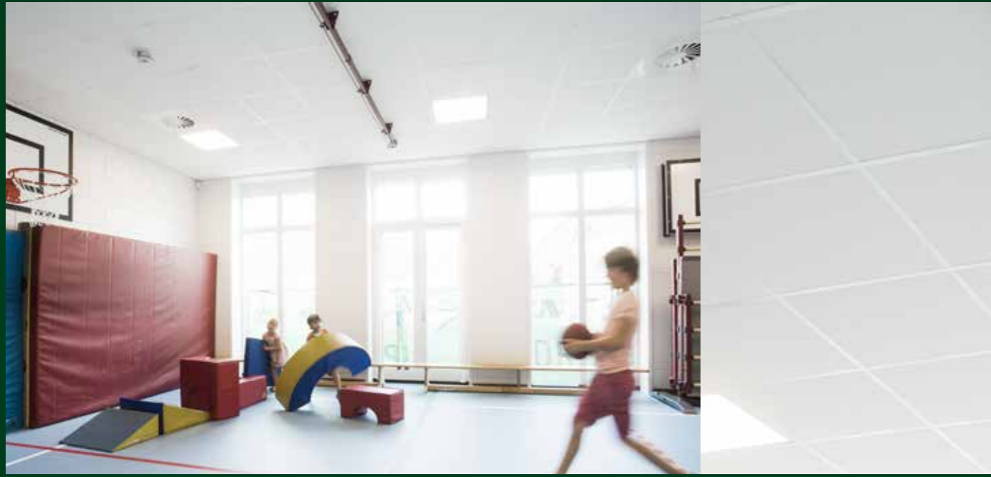
SUPER G A Visible grid system and impact bracing bars or clips to keep the panels in place.
